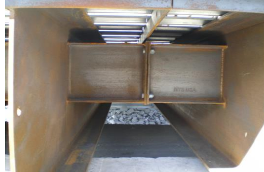
Center Diaphragms bolted together
