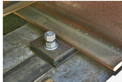
Bearing Plates field welded
