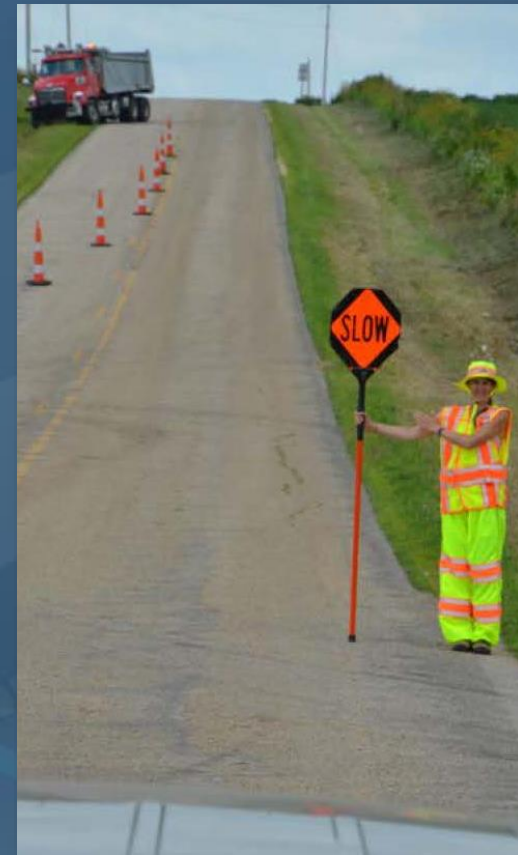
Releasing traffic into the open lane; standard drive lane
