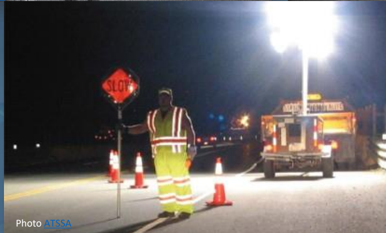
Photo: National Cooperative Highway Research Program Report 476
